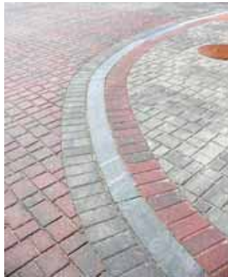
Changes in pavement texture, color and shape signal pedestrians and drivers alike to changes in grade and user priority.
