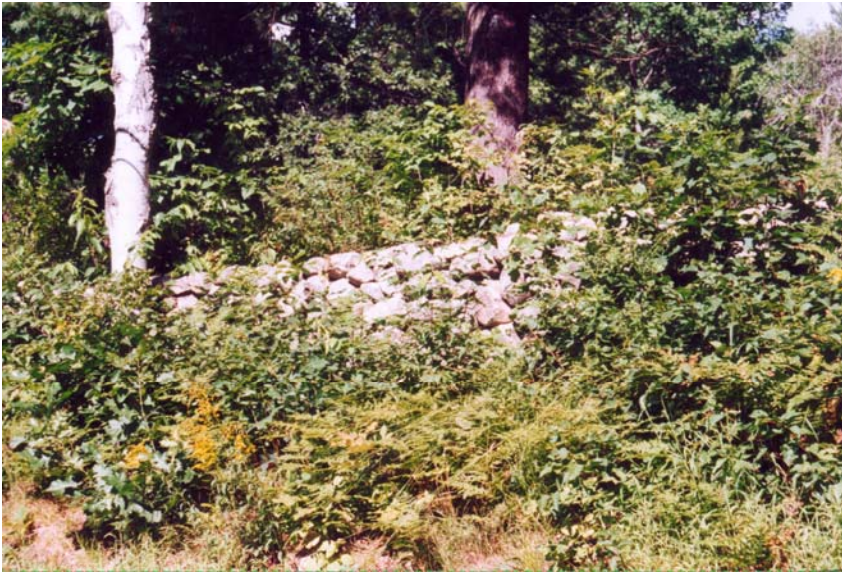
Young saplings and other successional growth obscure the original stone walls around Skyfields. Management recommendations include exposing and stabilizing the walls, but allowing succession in controlled areas for wildlife benefit.
